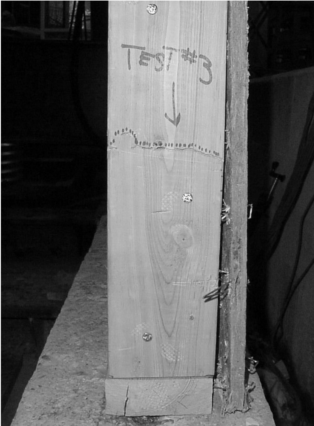
Figure 5.3. Panel 3 sheathing tearing and end wall stud crack.
