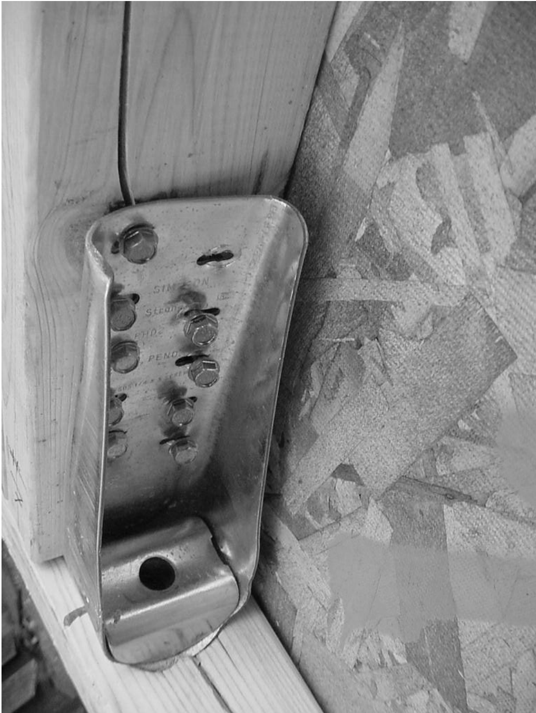
Figure 5.10. End-wall stud, hold-down, and sill failure panel 7.
