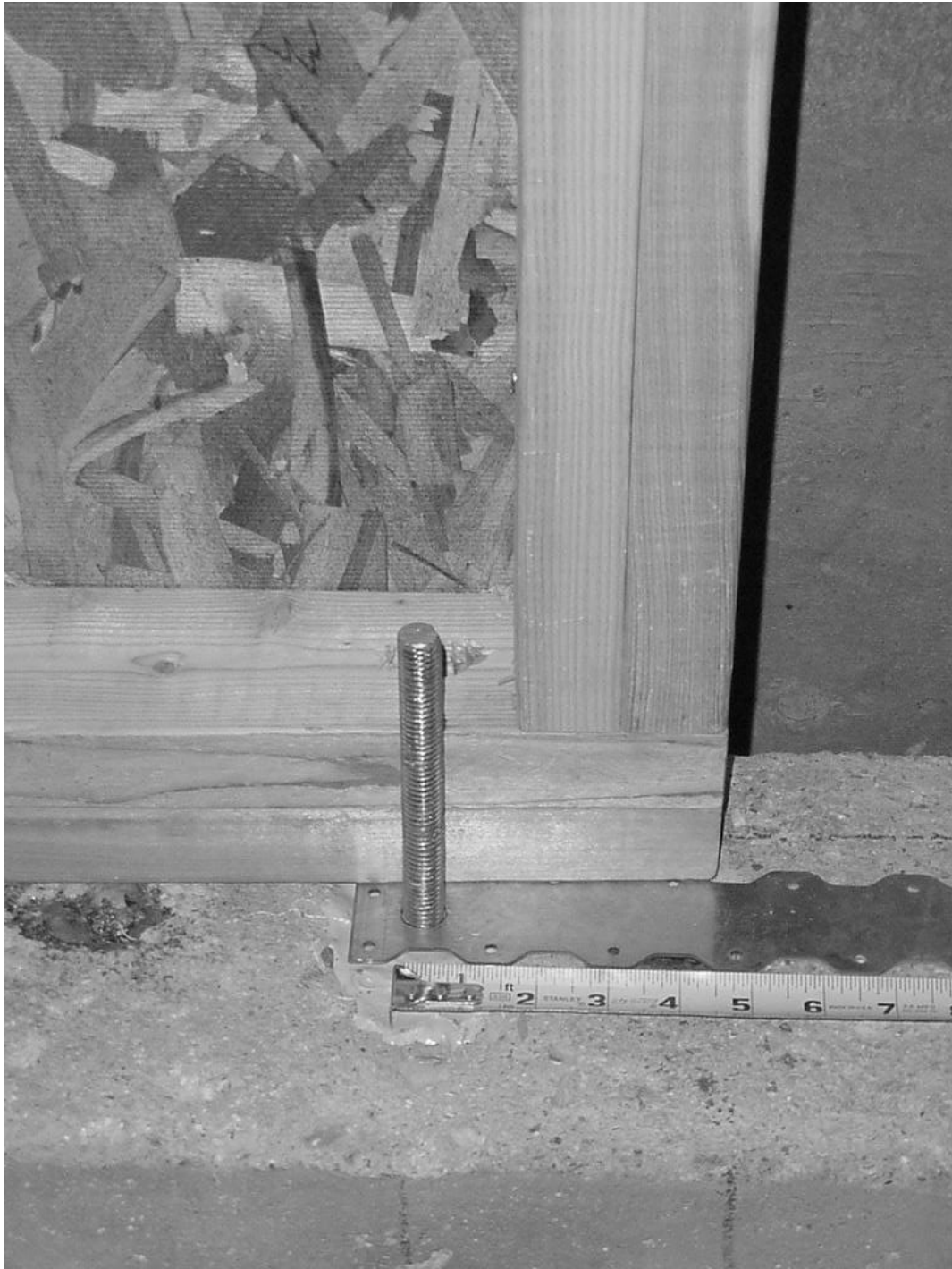
Figure 5.9. End-wall stud strap panel 7.
